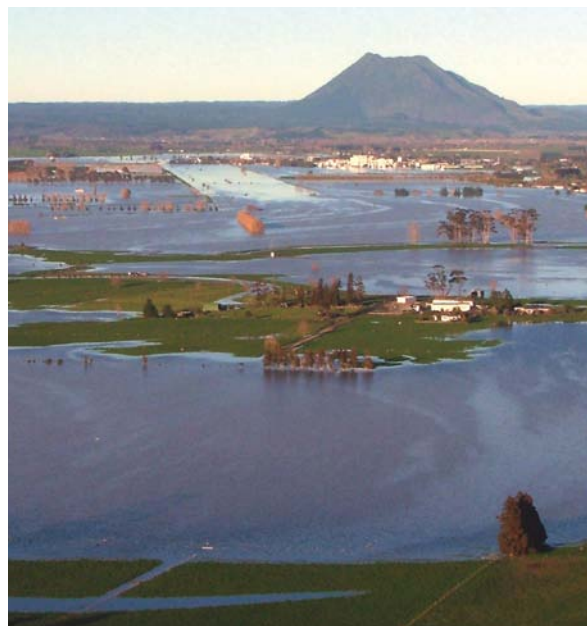
Flooding in the Bay of Plenty
